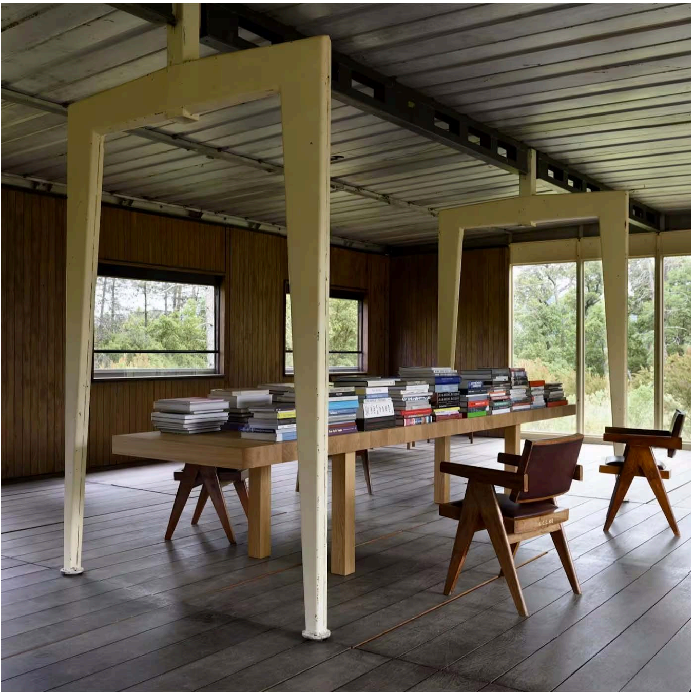
The interior with its hollow steel 'compass', an ingenious innovation that supports the ridge beam and stabilises the construction © Galerie Patrick Seguin
